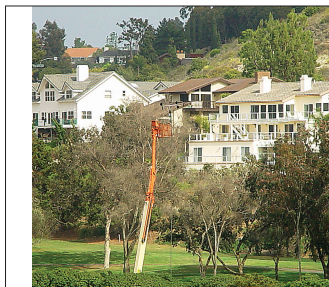
Figure 2.59 R/C crane for mounting receive antennas for wireless mics and cameras. Compound is below behind the trees.
